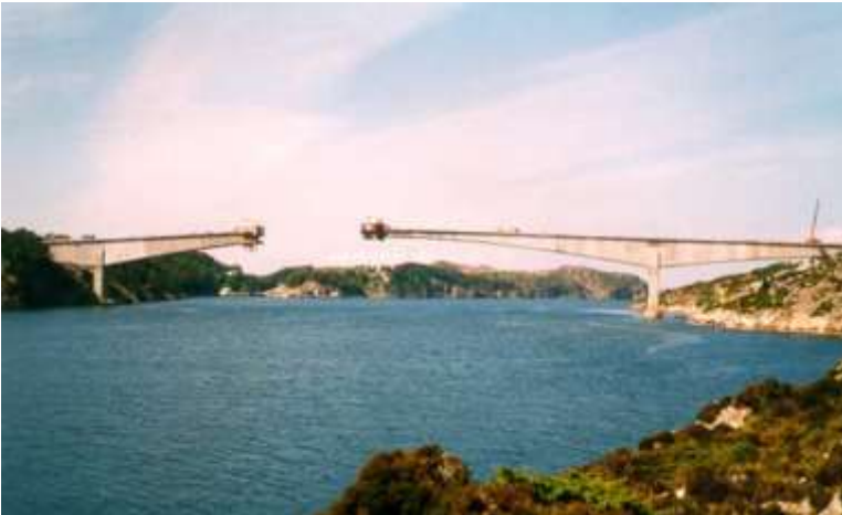
Figure 3. Stolma bridge in Norway, built of high-strength lightweight concrete
