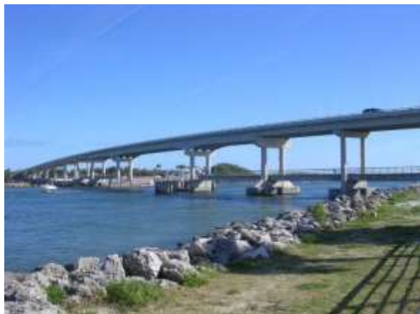
Figure 1. Sebastian Inlet Bridge
