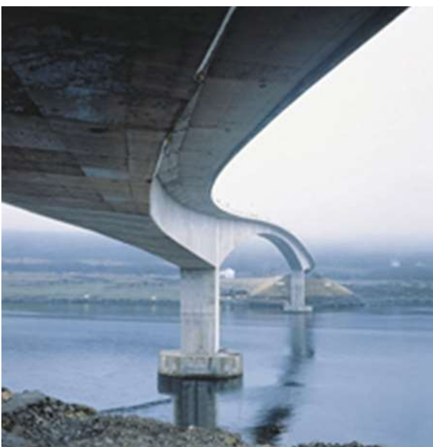
Figure 4. Stavset expanded clay concrete bridge in Norway (span between supports 150m) [44]
